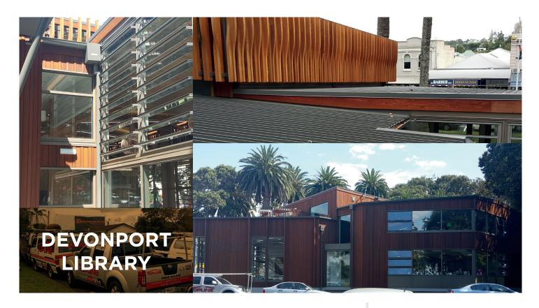
Devonport Library is a glulam portal structure with a cladding of vertical ship lapped cedar weatherboards which allows the library to blend in well with its park-like surroundings with windows framing the harbour views on the south and east sides of the building.
