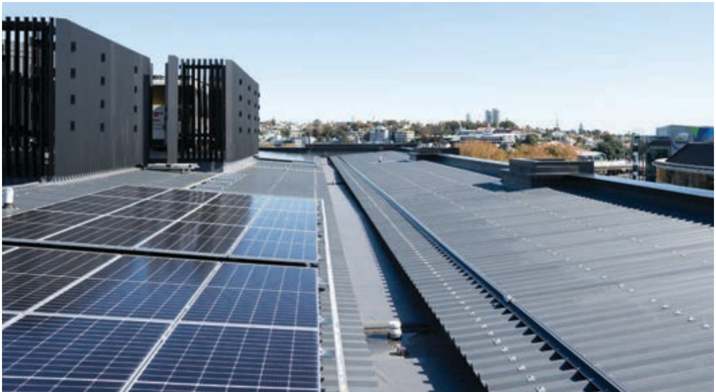
Te Aukati's roof incorporates a post-and-rail warm roof system installed across approximately 2,430m 2 , using 0.55g Magnaflow MSR Topdeck. The system was designed and installed to meet the performance requirements of a 6 Star Green Star building, supporting thermal efficiency, airtightness, and long-term durability. For more of their work visit www.toplineroofing.co.nz
